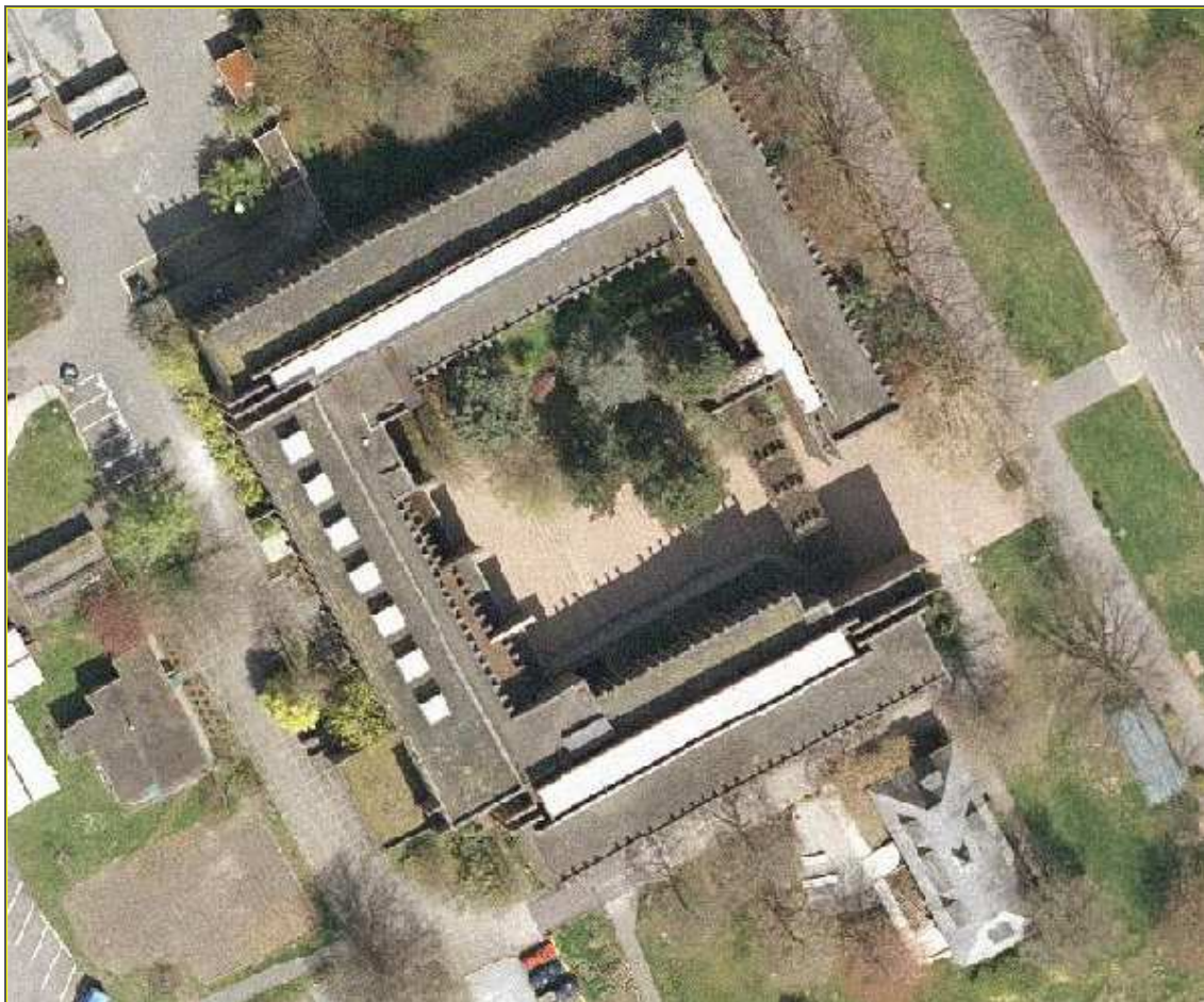
Figure 1 - Aerial View of the H.R. MacMillan Building
